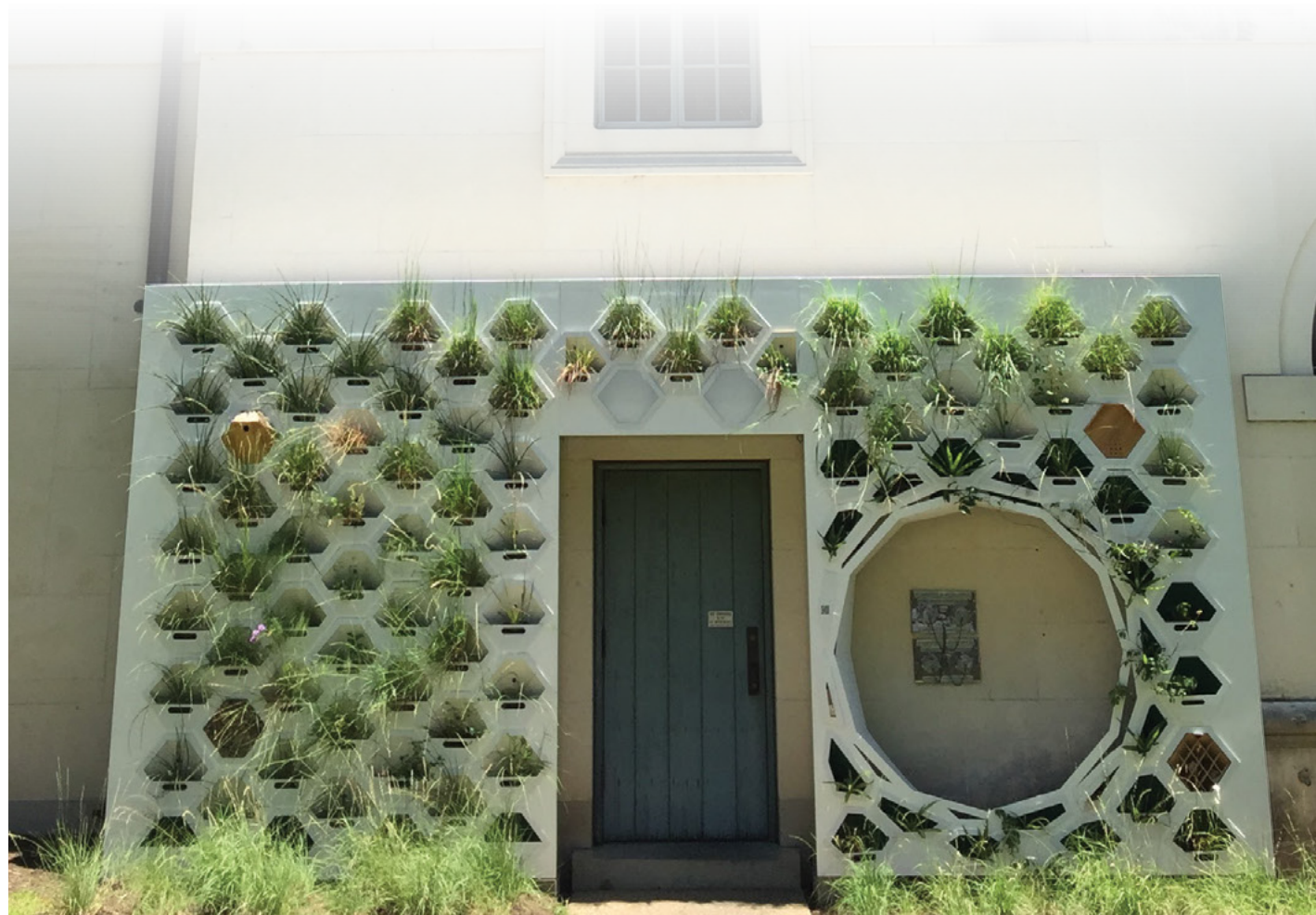
The School of Architecture's living wall attracts wildlife, helps cool the building, and serves as a natural air filter. Photo: Charlie Moore
