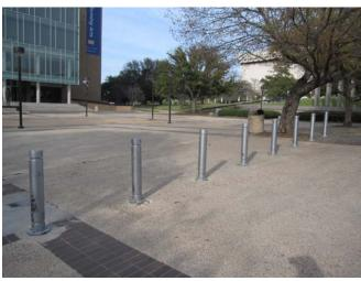
Where temporary vehicular access is required, bollards shall be removable or retractable
