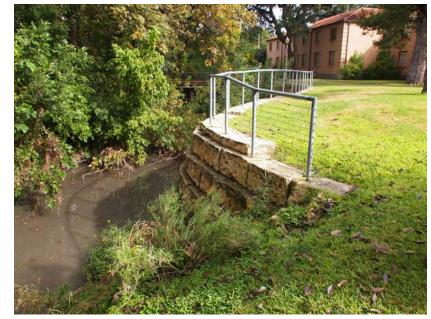
The creek channel shall be stabilized with limestone blocks in areas where the slope of banks exceed 6:1 in the floodplain.
