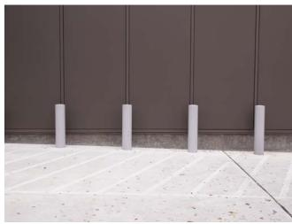
In service areas with low pedestrian use and visibility, simple pipe bollards with a powder coat paint finish of compatible color with the building are acceptable.
