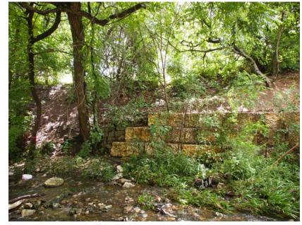
Unstable banks caused by urbanization and narrowing of the stream channel have been reinforced with a variety of limestone block walls.
