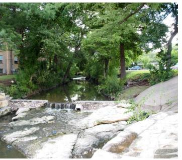
In stream structures should be removed to reduce the elevation of water profiles and avoid reverse hydraulic supercritical flows of floodwaters below the structures.
