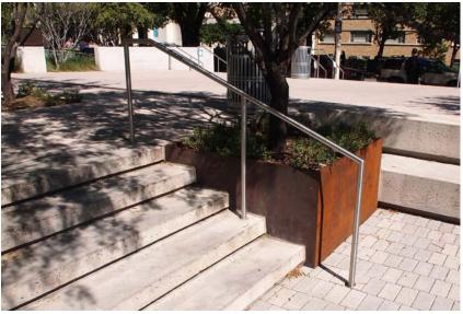
The simple profile of the stainless steel handrails at the Belo Courtyard fits in well in this contemporary setting, as well as in more traditional spaces.
