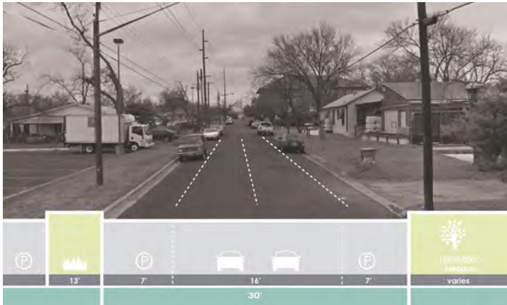
EXISTING CONDITION: LEONA STREET LOOKING NORTH
